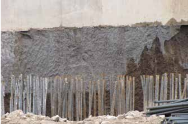
Fig. 24: Two kinds of cangagua under a concrete platform constructed for the station (Authors' archive)
