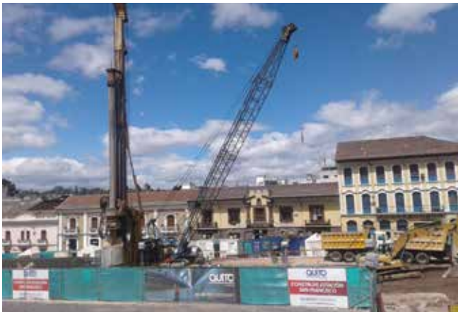
Fig. 20: After that, heavy machinery made perforations through cangagua structures for building piles for the station (Authors' archive)
