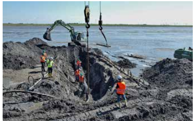
Fig. 5: Open trench for cable installation.
