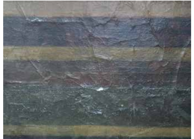
Fig. 5: The wall paintings of the Emperor's Hall, the main room of the Imperial Palatinate, show extensive flaking. Photo: Henning Frase
