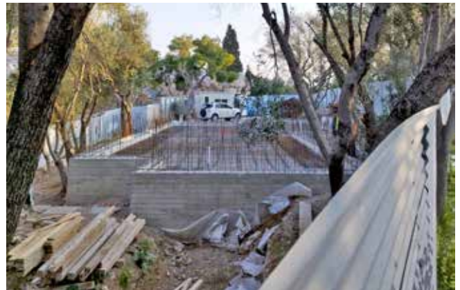
Fig. 6: The foundations of the new ticket office buildings, with vertical rods for the reinforcement of the walls. At the background the rock of the Areopagus. View from the south. (2024)
