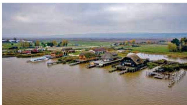
Fig. 4: The traditional reed-covered wooden houses on the lake shore, a defining feature of the cultural landscape and located in the core zone of the World Heritage, have all been totally destroyed in December 2020.
