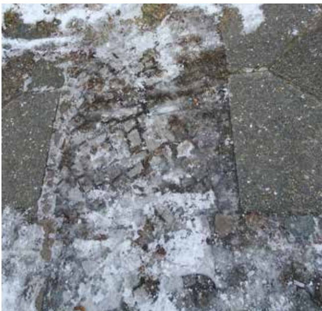
Fig. 4: Frozen rainwater spilled on the sidewalk from the gutters is a serious accident risk. Photo: Ute Scheub
