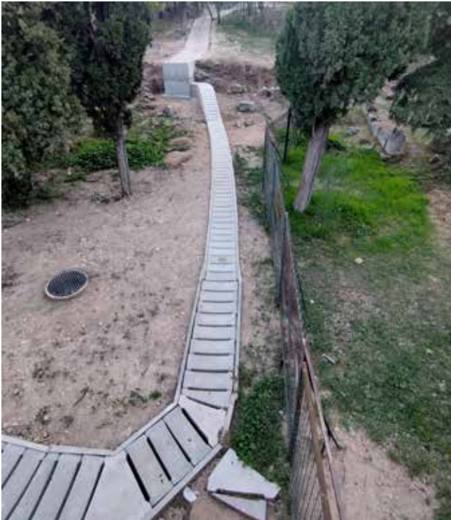
Fig. 3: Part of the dense network of massive drainage channels, built in reinforced concrete, spreading widely in the archaeological site below the Acropolis. (October 2022)
