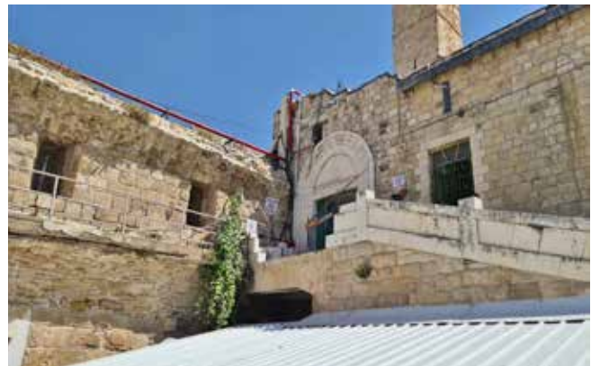
Fig. 5: Section of balustrade dismantled to make room for the bridge leading to the elevator.
