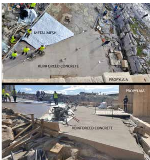
Fig. 1: Paving the rock to the east of the Propylaea. Above: The metal mesh spread on the white plastic sheet resting directly on the living rock. Below: To the right at the bottom of the picture, the thickness of the reinforced concrete resting on the living rock. (October 2020)
