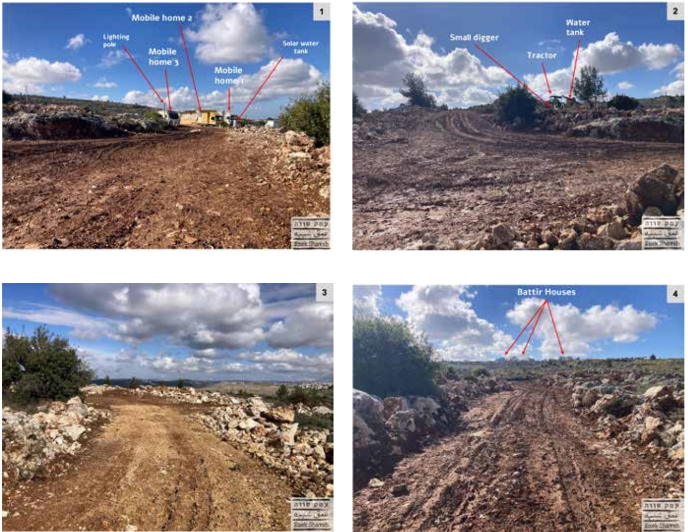
Fig. 5: The roads paved and the damage to the site. 1. Looking west on road 4. 2. Looking south at the intersection between 4 and 7. 3. Looking north at road 7, also visible is the northern access to the "flattened area". 4. Looking south at road 7. Road numbers as in Fig. 2.
