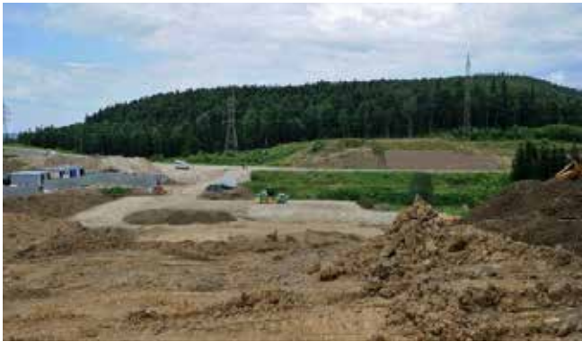
Fig. 5: Electric substation under construction.
