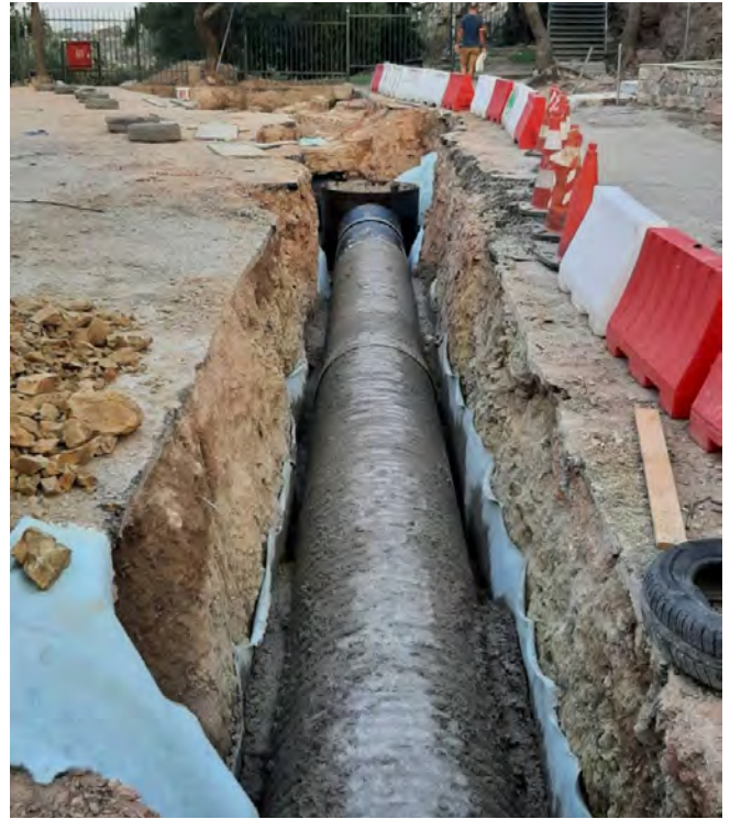
Fig. 4: Big plastic pipe buried to the south of the Areopagus, part of the drainage network. View of the ditch looking west. The big pipe is being encased in cement that will bear the fill to reach the surrounding ground level. (March 2023)
