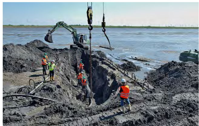
Fig. 5: Open trench for cable installation.
