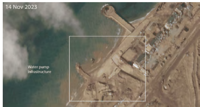
Fig. 12: Satellite image from 14 November 2023 of water pump infrastructure.
