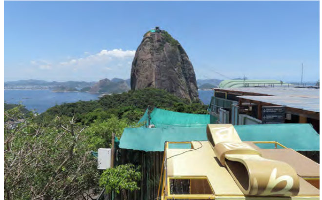
Fig. 12: The space once dedicated for the enjoyment of the view of the West Face of Sugar Loaf from the top of Morro da Urca is now partially hidden by large green sidings and canvas covers tightly fastened to anchors. Photo: André Ilha
