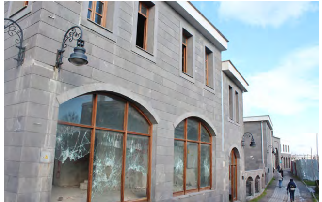
Fig. 9-10: Newly constructed buildings that have turned derelict due to disuse
