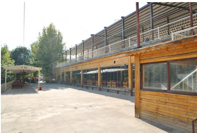
Fig. 17–18: Intense illegal construction surrounding the Tigris Bridge.
