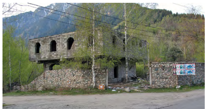
Fig. 2: Unfinished and abandoned building, Big Almaty Canyon, Ile-Alatau National Park (May 9, 2023).
