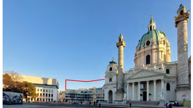
Fig. 4: St Charles Church and vicinity in 2024. The Wienmuseum with the new superstructure is on the left. The red lines show the planned 3-floor superstructure on top of the Winterthur office building.
