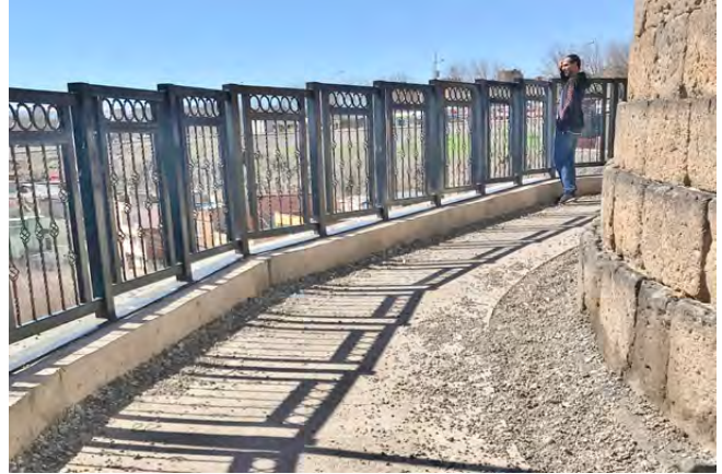
Fig. 2: Iron railing at the foot of the city wall
