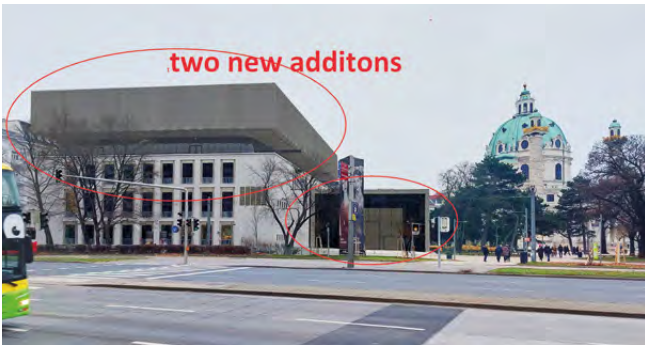
Fig. 3: St Charles Church and vicinity in December 2023. The Wienmuseum with the new superstructure and the new addition protruding towards the Ressel park.
