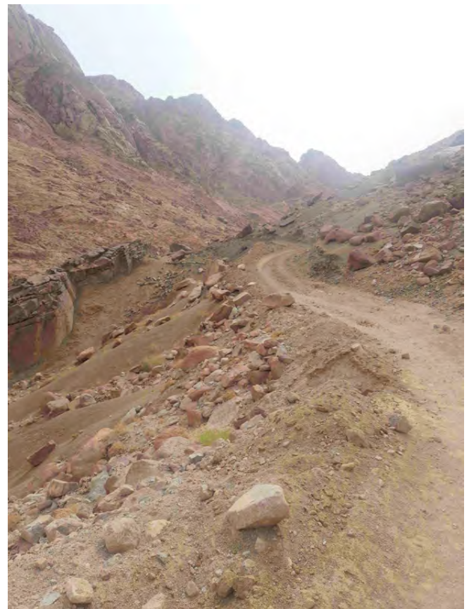
Fig. 7: New road cut through Wadi Hebran to the GTP. Photo: Anonymous
