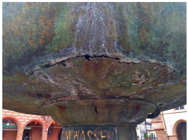
Fig. 9: The crack in the upper bowl of the market fountain. Photo: Henning Frase
