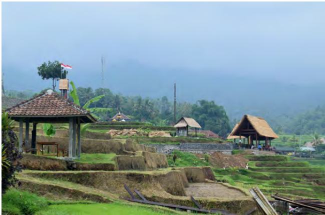
Fig. 4: New construction site in Subak Jatiluwih.
