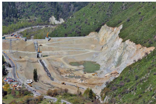
Fig. 4: New construction on the riverbank, Kimasar Canyon, Ile-Alatau National Park (May 2, 2023).
