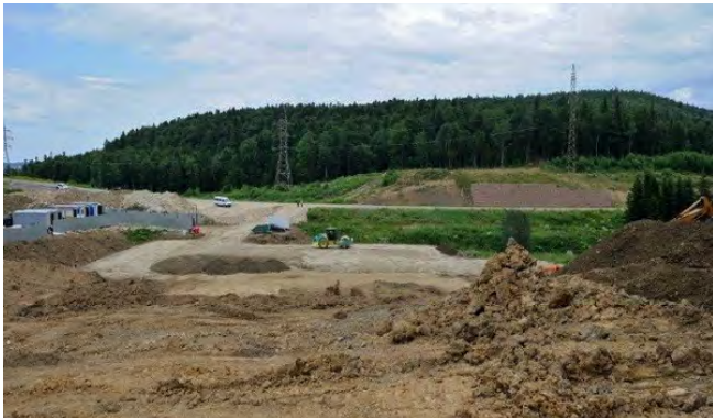
Fig. 5: Electric substation under construction.
