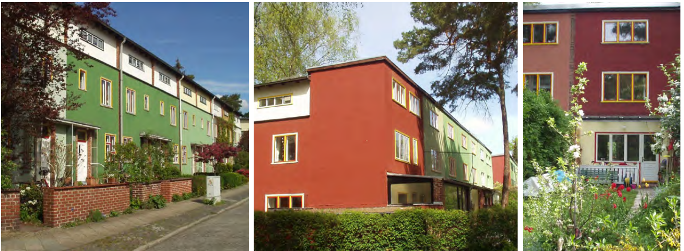
Fig. 1-3: Buildings in the Waldsiedlung Zehlendorf.
