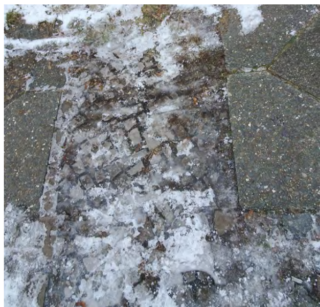
Fig. 4: Frozen rainwater spilled on the sidewalk from the gutters is a serious accident risk. Photo: Ute Scheub
