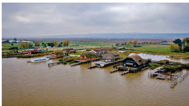
Fig. 4: The traditional reed-covered wooden houses on the lake shore, a defining feature of the cultural landscape and located in the core zone of the World Heritage, have all been totally destroyed in December 2020.
