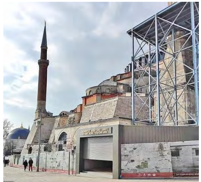
Fig. 8: Temporary Entrance Structure of the Visitor Area.
