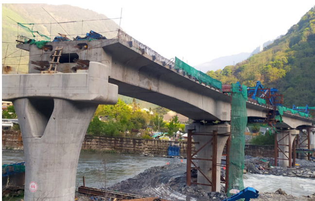
Fig. 7: The high-speed train from Dujiangyan to Mt. Siguniang under construction crosses the WH property, but may not impact the core and buffer zones of the GP NP. Photo: Martin Lenk, 27.4.2024
