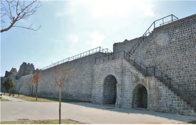
Fig. 4: Railings built on the city walls between Yedikardeş Bastion numbered 41 and the bastion numbered 40. Photo: Pinar Can, DKVD Diyarbakır City Archive, 5.03.2025
