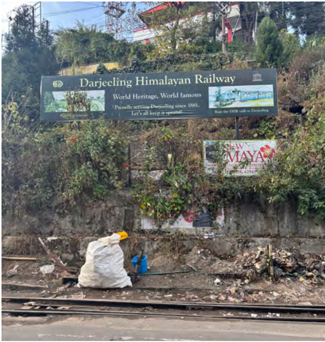
Fig. 5: Garbage dumped on the tracks at Kurseong.
