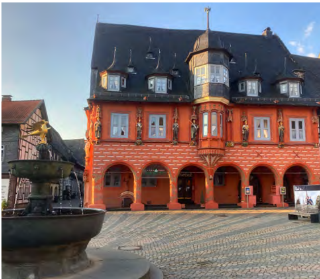
Fig. 1: The change of ownership of the important Hotel Kaiserworth, shown here, and Brusttuch buildings has brought great relief to the residents of Goslar's old town. The sale of the buildings will help to revitalize the entire area around the market square and the market church.
