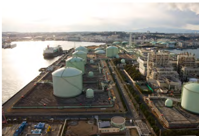
Fig. 1: The Negishi LNG Terminal, Japan, is an example of large-scale LNG infrastructure. It helps visualize the type of industrial development these projects would involve in the Gulf of California. Its capacity is also significantly smaller than that of proposed terminals like Vista Pacífico LNG or Saguaro Energía
