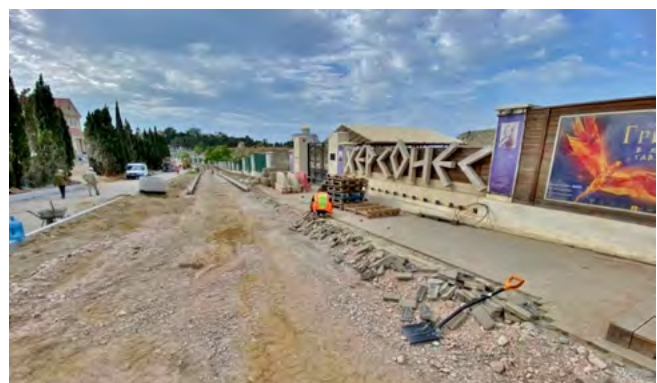
Fig. 2: Construction in Drevnia street in the site of Tauric Chersonesos, 2024.
