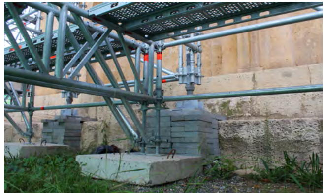
Fig. 3: Church of the Virgin, Scaffolding concrete and stone slab supports on ground and church structure, October 10, 2024. Photo: Manon Liluashvili
