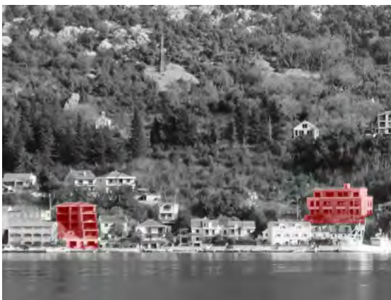
Fig. 7: Another example from Dobrota, below the Church of St. John, where a building under construction with a ground floor and four floors completely surpasses all existing structures. The building at the right, was built in the past two years on cultivated terraced landscape with very ancient oak trees, which have been removed. This building represents an example of structure permitted under the SUP.
