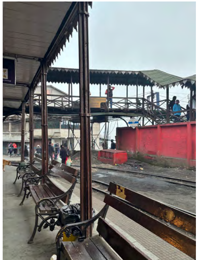
Fig. 4: Maintenance and upkeep leave much to be wished for, here at the Ghum Railway station.
