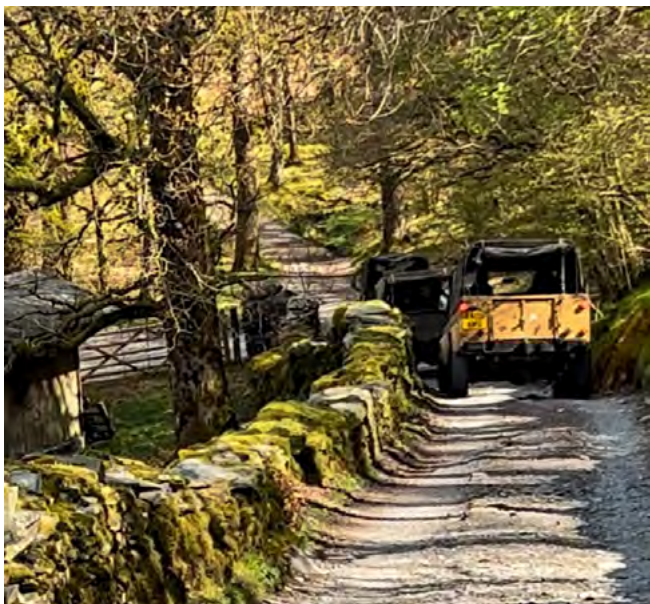
Fig. 1: 4x4 vehicles on Hodge Close green lane. Photo: Lake District Green Lanes Alliance
