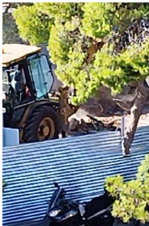
Fig. 9a. 9b: Two successive stills from a video showing a mechanical excavator at work, at the area destined for the new souvenir shop. (2023)
