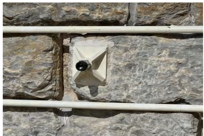
Fig. 10a: "Consolidation" of the Agrippa Pedestal. Prestressed rods, framing the periphery of the course on top of the foundation. Two prestressed rods inserted in cylindrical holes that are straight through and enter and exit on the external surfaces of the course. (2023)
