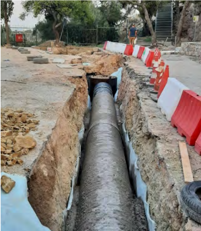
Fig. 4: Part of the dense network of utilitarian infrastructure. A big plastic pipe buried to the south of the Areopagus, part of the drainage network. View of the ditch looking west. The big pipe is being encased in cement that will bear the fill to reach the surrounding ground level. (March 2023)
