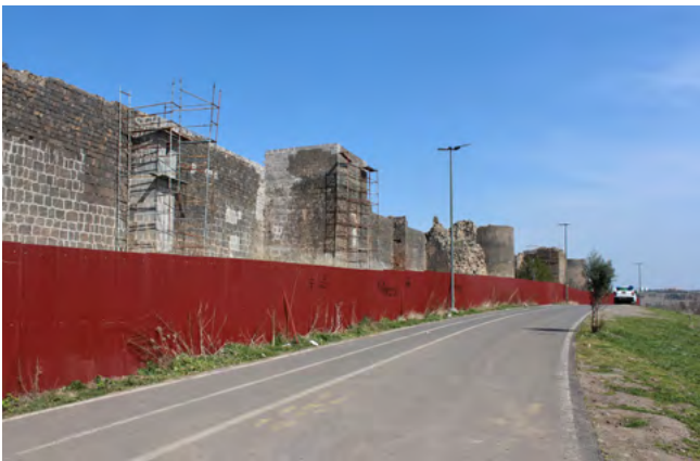
Fig. 1: The road that runs along the bottom of the city walls is open to vehicle traffic. Photo: Pinar Can, DKVD Diyarbakır City Archive, 5.03.2025
