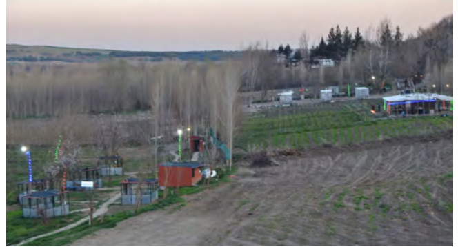
Fig. 9: Illegally built structures in Hevsel Gardens and operated as cafes.
