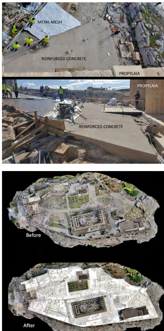
« Fig. 1: Paving the rock to the east of the Propylaea. Above: The metal mesh spread on the white plastic sheet resting directly on the living rock. Below: To the right at the bottom of the picture, the thickness of the reinforced concrete resting on the living rock. (October 2020)
