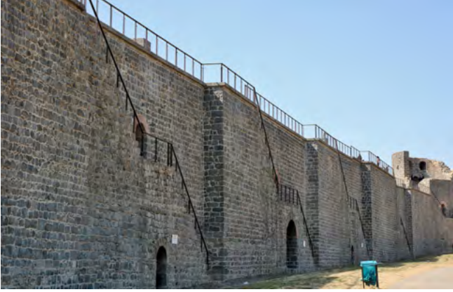
Fig. 3: Railings built on the upper parts of the walls of İçkale. Photo: Pinar Can, DKVD Diyarbakır City Archive, 5.03.2025
