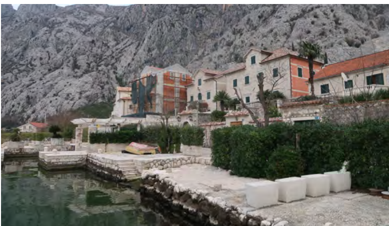
Fig. 10: In the north part of Ljuta, at the first row along the coast, a newly constructed building, interpolated into a row of traditional structures, exceeds the highest traditional building - a small palace - by an entire floor. The approval document for the project states that the building has a three floors P+1+Pk (three visible levels: ground floor, first floor, and attic). However, it is evident that the floor count was not calculated from the coastal road elevation, which should have been a requirement, and the attic was constructed as a full-height floor.
