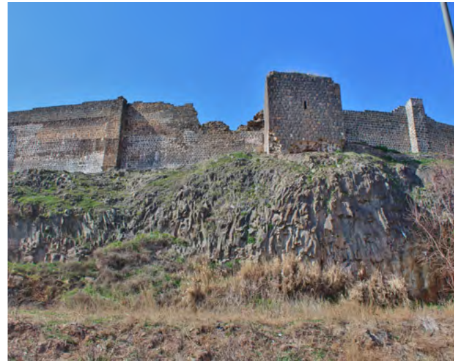
Fig. 2: Restoration of the eastern city walls. See also Fig. 1.
