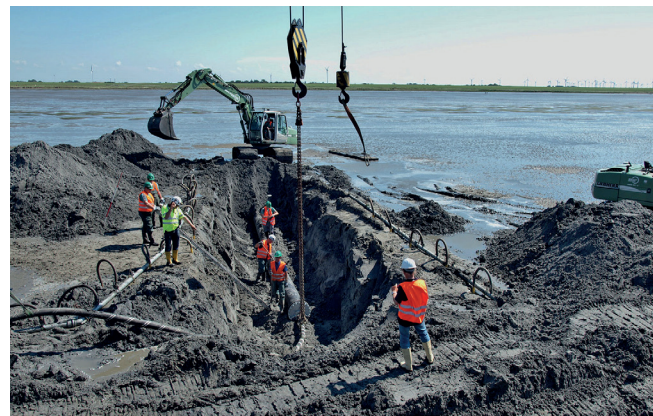
Fig. 5: Open trench for cable installation.
