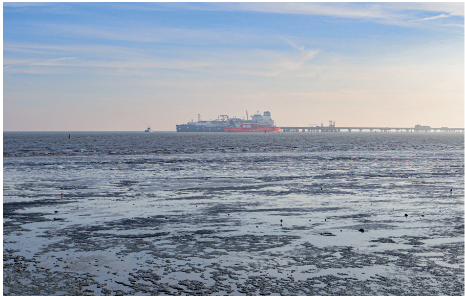
Fig. 2: In Wilhelmshaven, the floating LNG terminal Höegh Esperanza operates with negative impacts on the Wadden Sea including chlorine and wastewater discharge.
