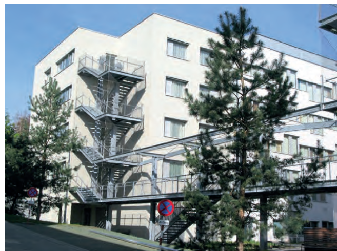
Fig. 10: VAMED building. Photo: Christian Schubböck
