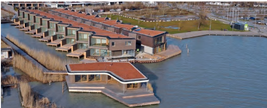
Fig. 3: Project “Am Hafen” in Neusiedl am See (left) and completed buildings in February 2020 (right). Graphic and photo: www.amhafen.at/de/Baustelle
