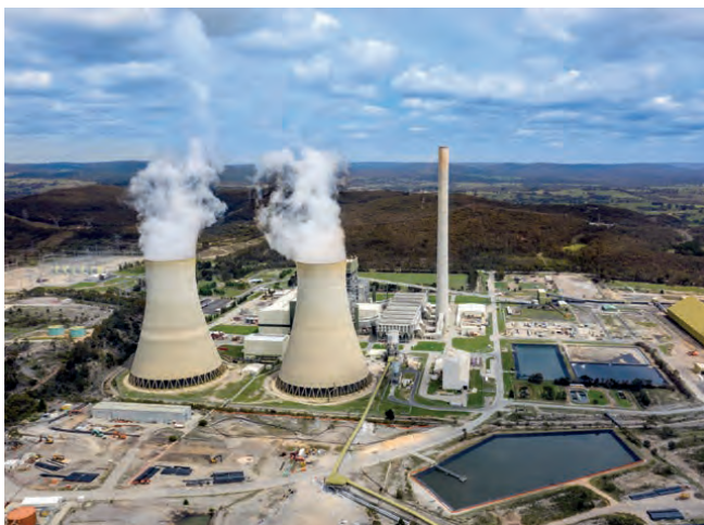
Fig. 4: Mount Piper coal power station in Portland, NSW. Photo: Getty Images/ mikulas
