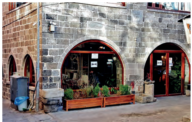
Fig. 9–11: A restaurant in Suriçi built with basalt stones taken from the city walls, 18 December 2019
