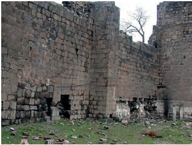
Fig. 1: Mardin Gate Walls, 20 February 2002
