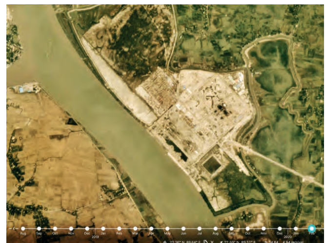
Fig. 2: The Rampal coal-fired power plant construction site, February 2020.
