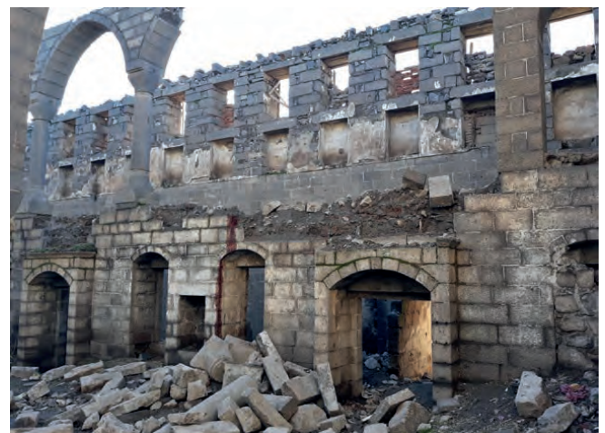
Fig. 7: Destroyed part of the Surp Sarkis Church with Western entrance, 18 December 2019
