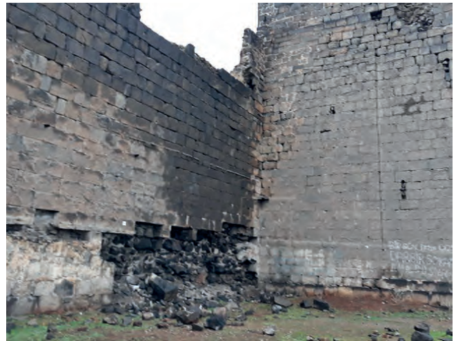
Fig. 2: Mardin Gate Walls, 27 December 2019
