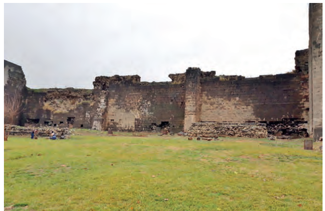
Fig. 4: Mardin Gate Walls, 27 December 2019
