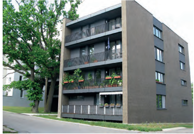
Fig. 7: GESIBA residential building (1). Photo: Christian Schubböck
